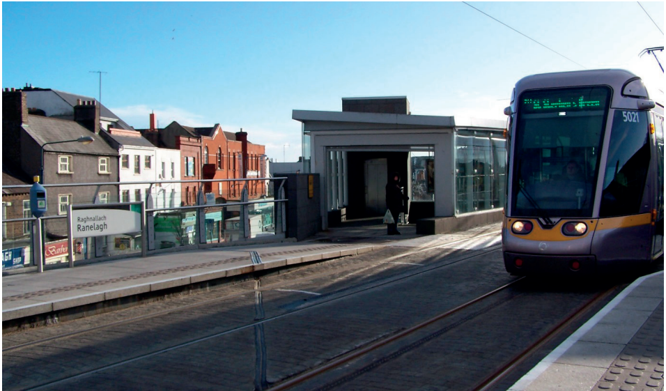
Pict. 6. Tram route in Dublin run on the flyover
